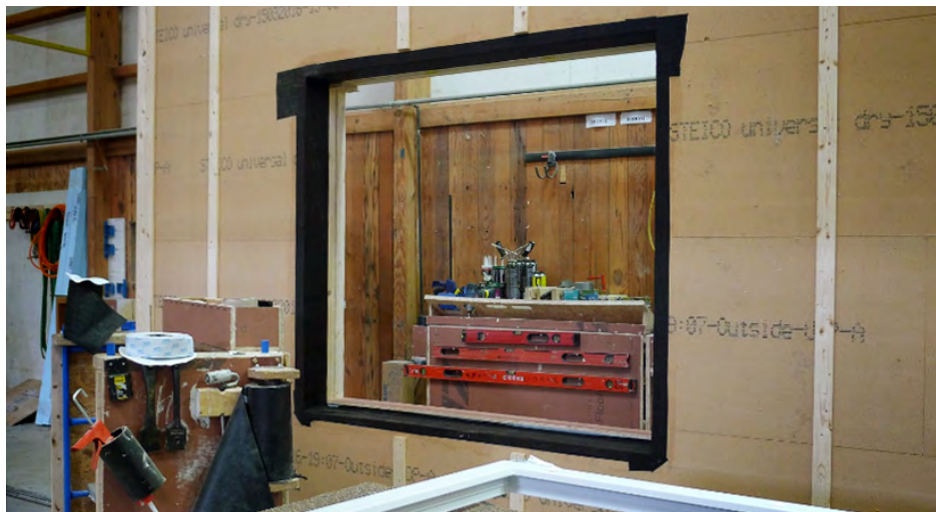
Air sealing a window rough opening
