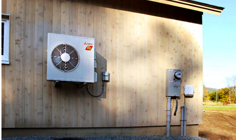
wall-mounted compressor
