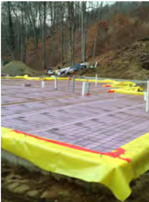
Slab insulation and vapor barrier
