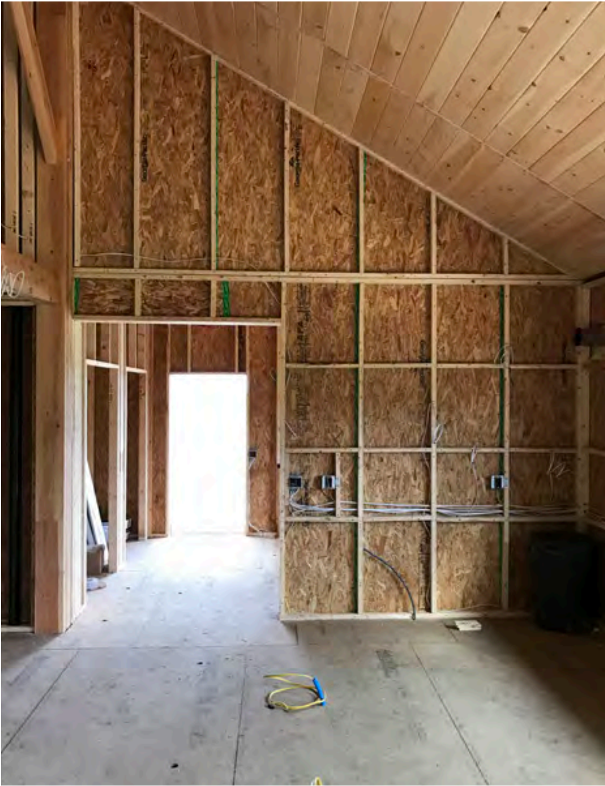
Mechanical, Electrical and Plumbing (MEP) Rough In
