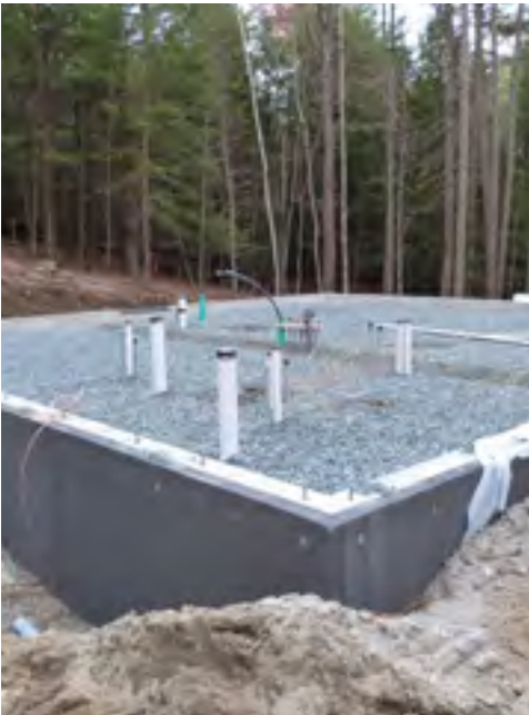
Subslab preparation
