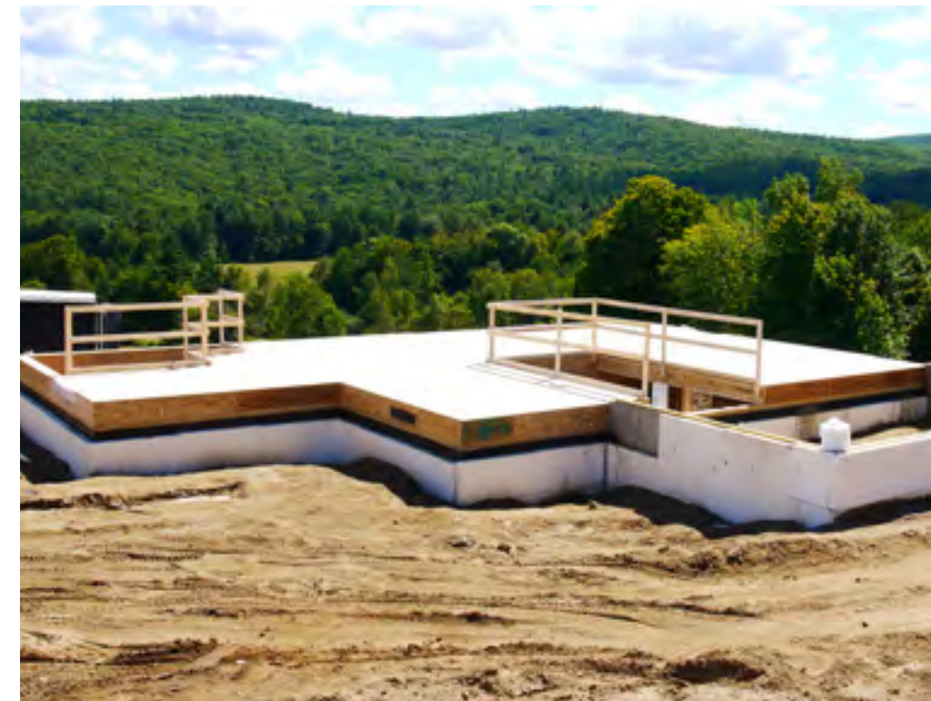
Completed first floor deck framing
