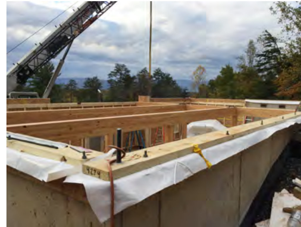
Columns and beams to support first floor framing
