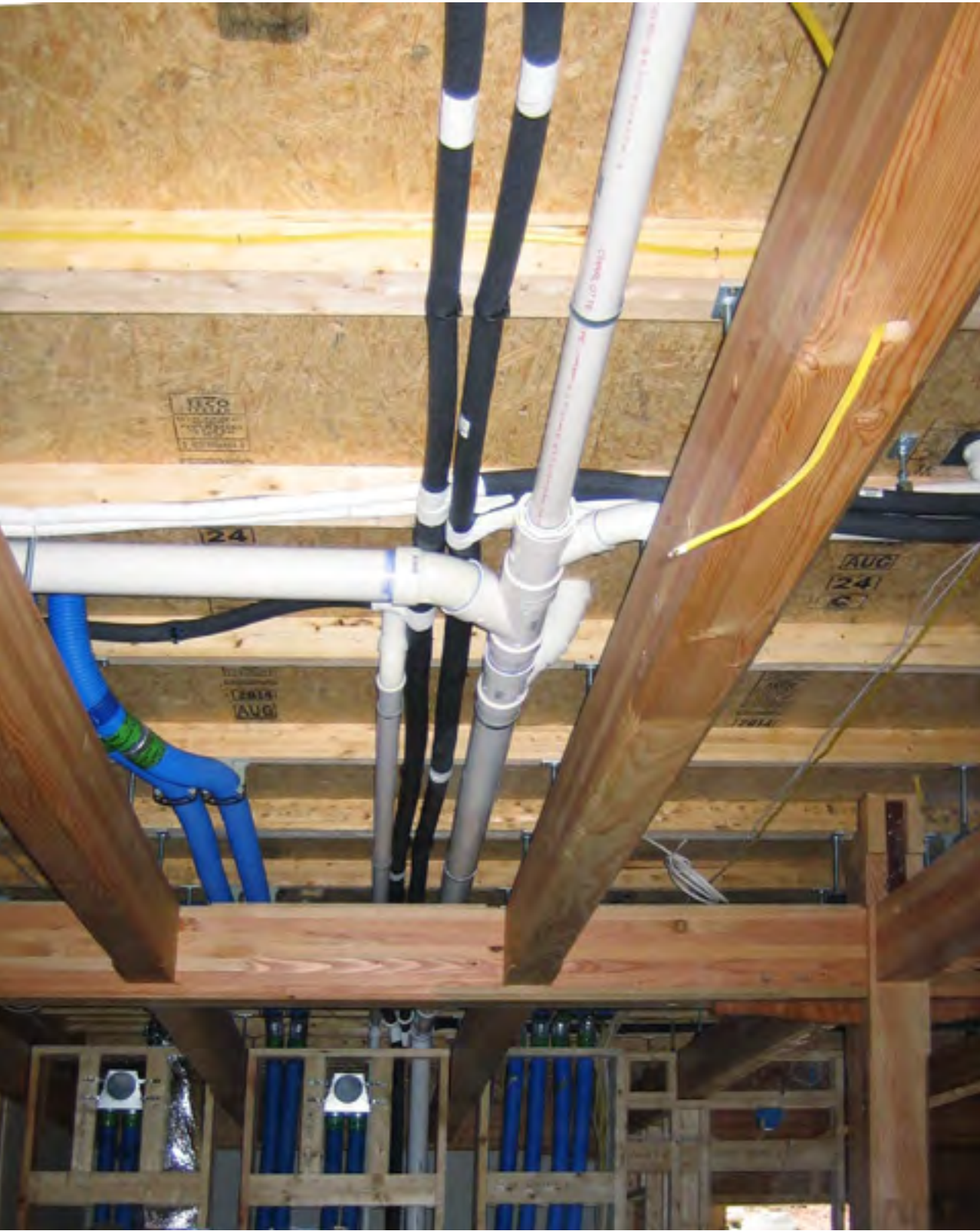
Mechanical, Electrical and Plumbing (MEP) Rough In
