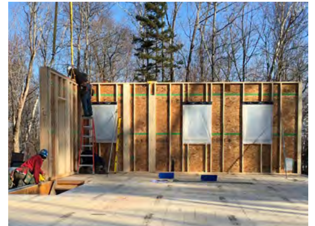
Setting the first floor walls
