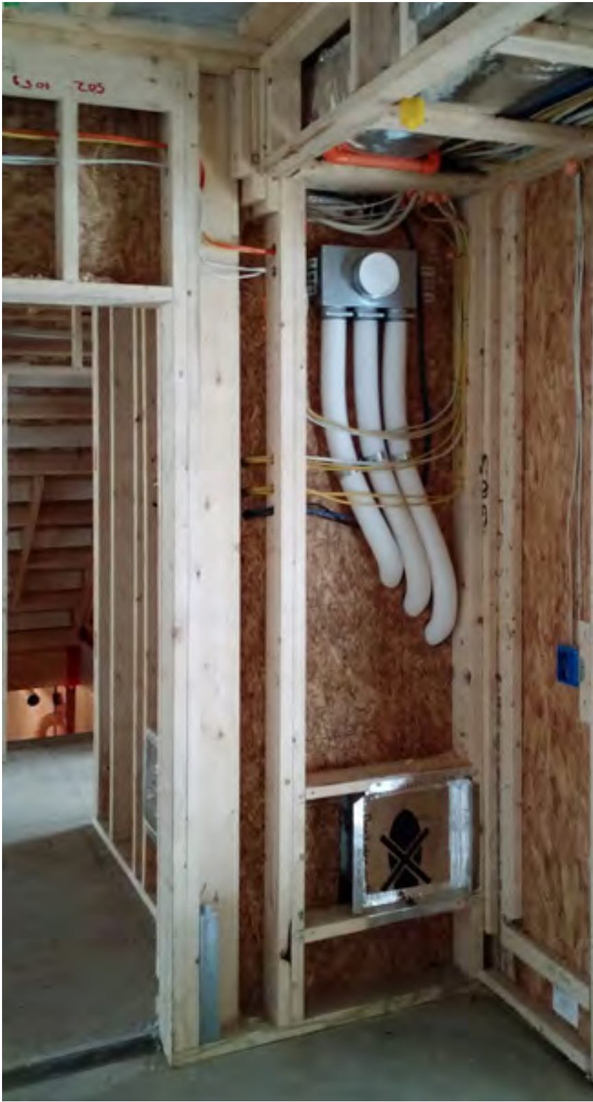
Mechanical, Electrical and Plumbing (MEP) Rough In
