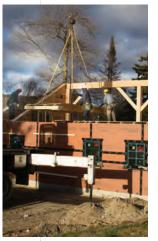
The Unity Homes 'Montage' process begins when we deliver the building component bundles to your site. The bundles are unwrapped from their weather-protective covering and each panel (floor, wall or roof) is then lifted into place in a sequence optimized for efficiency. In just a few days your home will take shape and be weathertight. Although we have built many homes in this way, the speed of the process still impresses us. We are confident that you'll be impressed tool
